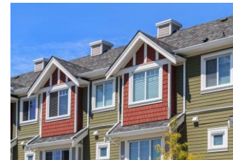
Permanent Supportive Housing
